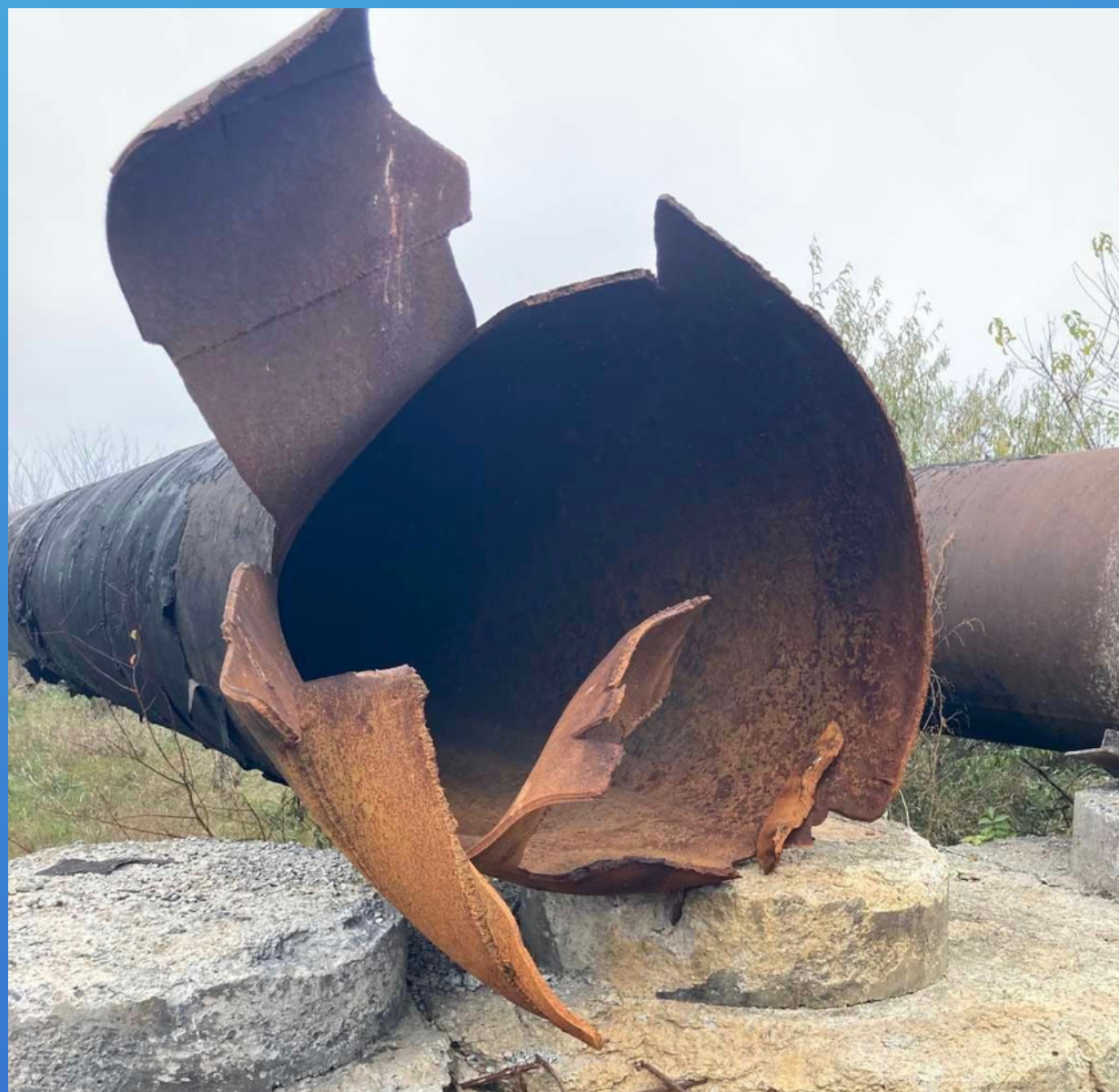
MAIN WATER PIPELINES
