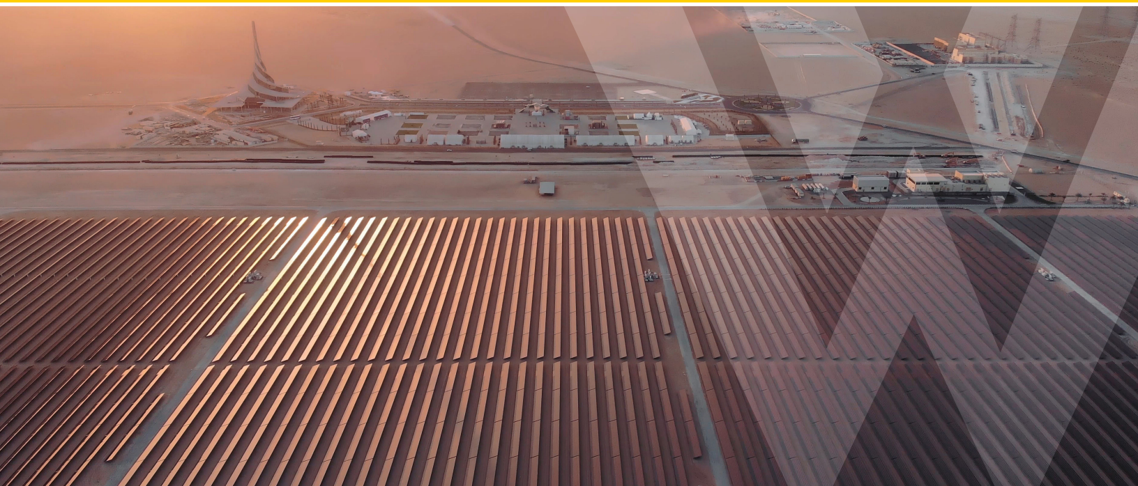
Mohammed bin Rashid Al Maktoum Solar Park in Dubai, UAE (SkyMediaPro / Shutterstock)
